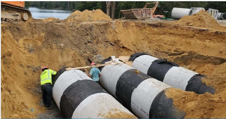
Tri-State Utilities installs new triple 54" RCP under Five Forks Road
