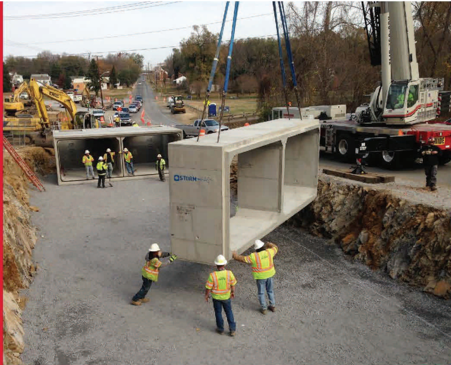
E.C. Pace Co., Inc. installs double 12x8 STORM-PASS® system in one day
