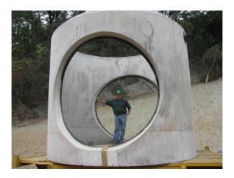
The 72" diameter reinforced concrete pipe was produced with rubber gasket joints and requires field testing in accordance with ASTM C1103. The 126" diameter precast manholes were produced with ALOK pipe connections to receive the 72" diameter concrete pipe. Construction is expected to continue through most of 2011.
