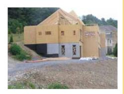
windows and doors. The single-piece corner sections are monolithically poured for exceptional strength. Most foundations can be set in a single day and provide a wall 10 times stronger than block or poured-on-site walls. The foundation is laid with the same technology used to make precast concrete bridges. This technology
