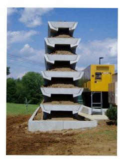
The Evergreen Wall can be a free standing sound wall or a retaining wall. When planted, its ability to promote plant growth makes it a very environmentally friendly alternative to other sound and retaining wall systems.
