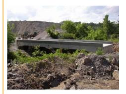
Final design also included a three-inch asphalt overlay. The resultant maximum loads were approximately 30.5 kips per linear foot vertically and 15.5 kips per linear foot horizontally, far exceeding normal loading for standard highway bridges.
