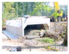
The OmegaSpan is quick to set and lasts longer than the corrugated metal arch.
