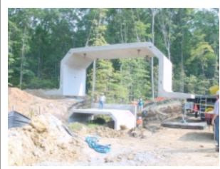
The OmegaSpan is a three-sided bridge structure that requires no cast-in-place footings.
